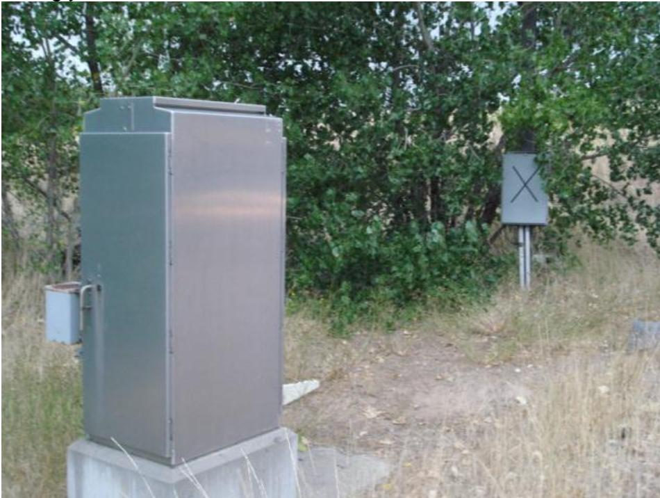
The large cabinet in front is apparently the control box for the UDOT traffic camera on top of a tall pole just out of sight to the left (see below). The smaller control box marked conveniently with an 'X' is what I had been looking for. UDOT must use the same data/audio link for both the camera and AM transmitter.
