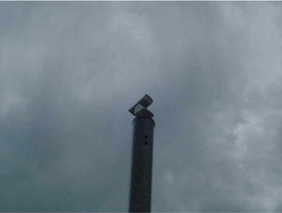
The AM transmitter is controllable up to 10 watts depending on the frequency. UDOT endeavors to keep the range under five miles<sup>1</sup>. This one is powered by 110 VAC, but can be solar powered. Portable units are solar powered.
