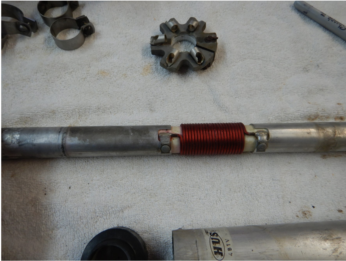
Figure 2: Examples of more corrosion found inside the traps
