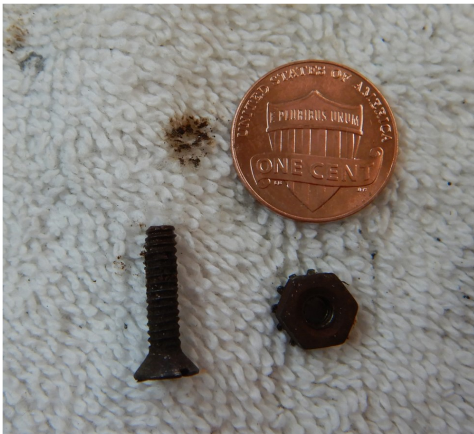
Figure 6: These are the worst examples – This one had enough of a slot left I could unscrew it. The other five screws had to be cut with a chisel
