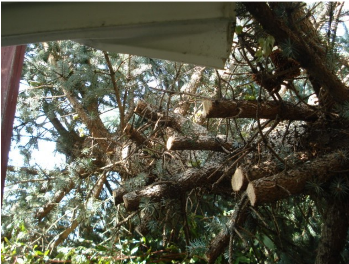
This is what I have to cut through. Trunk is about a foot thick.
