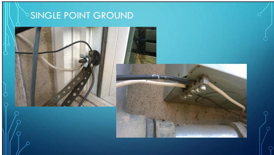
This slide shows the outside of my shack. The white and black wires go to the single point grounding bus on the electrical service panel. The other wires go to additional ground rods that I added. The single point grounding buss on the service panel also connects to other ground rods. I will be adding one additional ground rod to my system and replacing all exterior grounding wire with #6 wire. I currently have 4 ground rods outside my shack.
