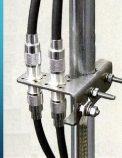
Use a Grounding Block. However this method does not ground the center conductor.
