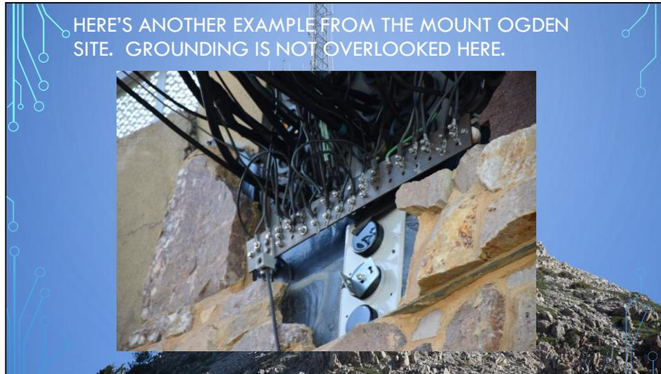
This picture is of the entry point into the Mount Ogden building. On the inside of the building EVERY coax line is protected with a Lightning Arrestor. They do not overlook lighting protection here. It's understood that a lightning strike is a certainty. Through the use of proper grounding they have turned a high probably risk into a low impact event. This is lighting protection done right.
