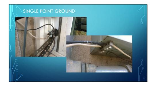
This slide shows the outside of my shack. The white and black wires go to the single point grounding bus on the electrical service panel. The other wires go to additional ground rods that I added. The single point grounding buss on the service panel also connects to other ground rods. I will be adding one additional ground rod to my system and replacing all exterior grounding wire with #6 wire. I currently have 4 ground rods outside my shack.
