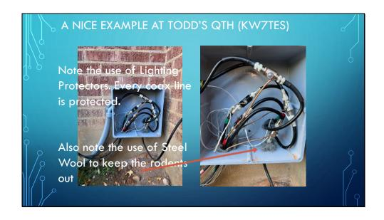
This is a good example of protecting your shack from surges from entering the shack. Todd has installed a lighting Arrestor on every bit of coax in his shack.
