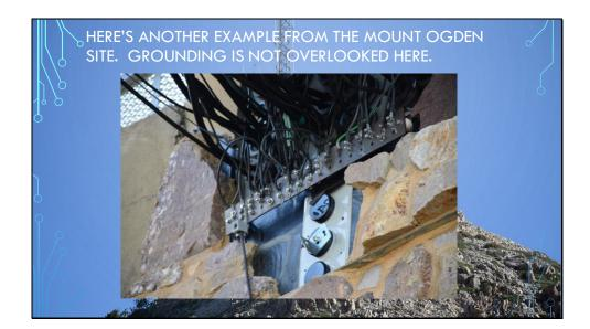
This picture is of the entry point into the Mount Ogden building. On the inside of the building EVERY coax line is protected with a Lighting Arrestor. They do not overlook lighting protection here. It's understood that a lighting strike is a certainty. Through the use of proper grounding they have turned a high probably risk into a low impact event. This is lighting protection done right.
