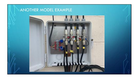
This is a model example. Note how the rotator wires are also protected.
