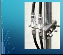
Use a Grounding Block. However this method does not ground the center conductor.
