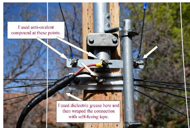
Figure 2: Using Dielectric grease, self-fusing tape, and anti-oxidant compound
